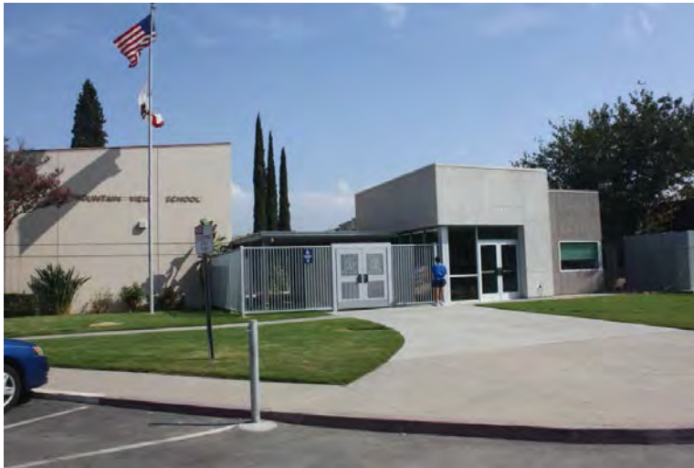
Completed Administration Addition
