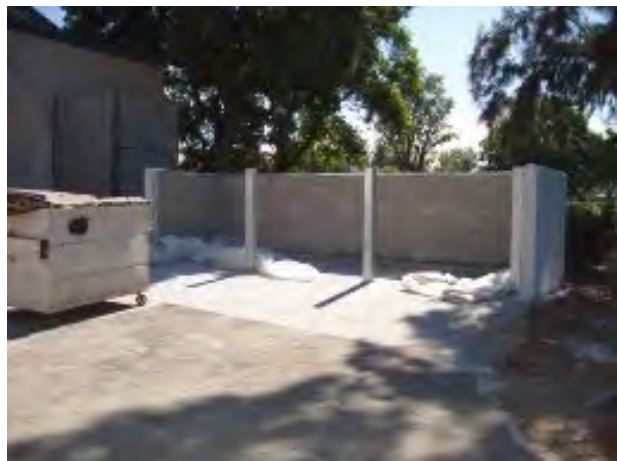
New Trash Enclosure
