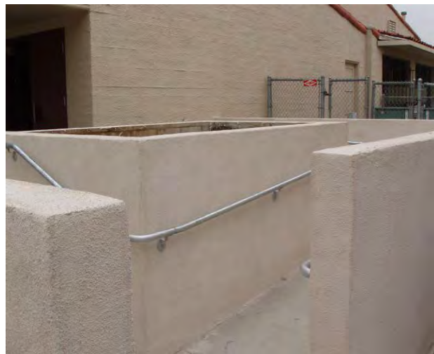
Outside MPR New ADA Ramp/Stairs
