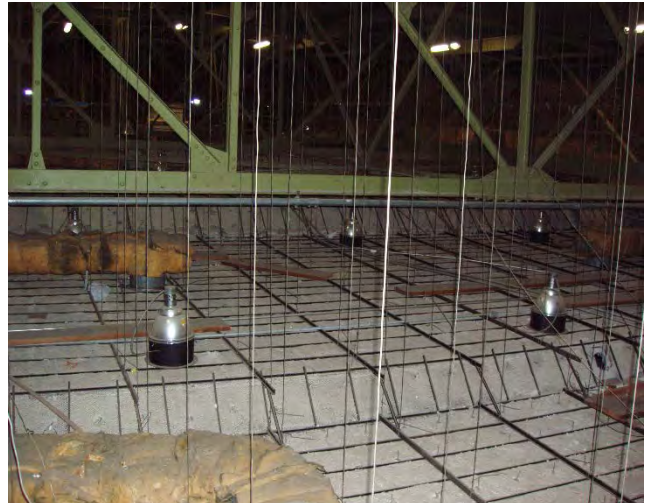
Suspended Plaster Ceiling
