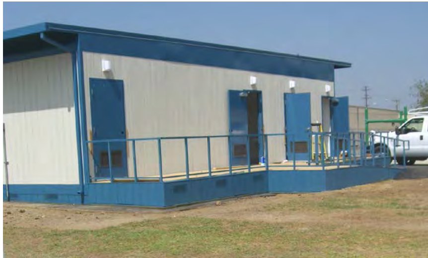
Completed Accessible Restroom
