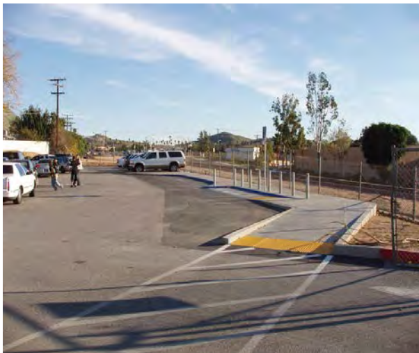
New Accessible Drop-Off Area
