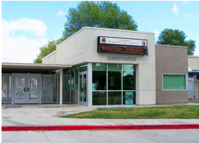
Administration Office Addition
