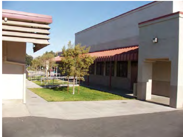
Landscaping at the New Multi-purpose Room
