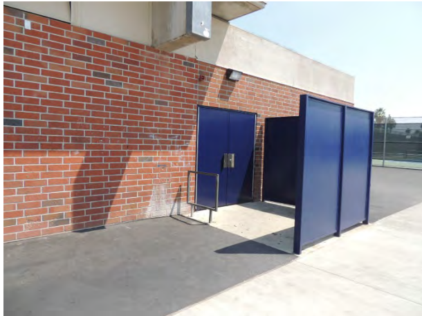
New Locker Room Plywood Modesty Panels
