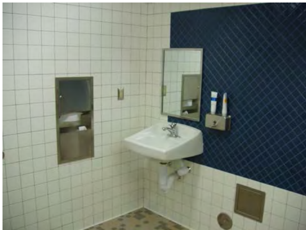
Completed Restroom Renovation
