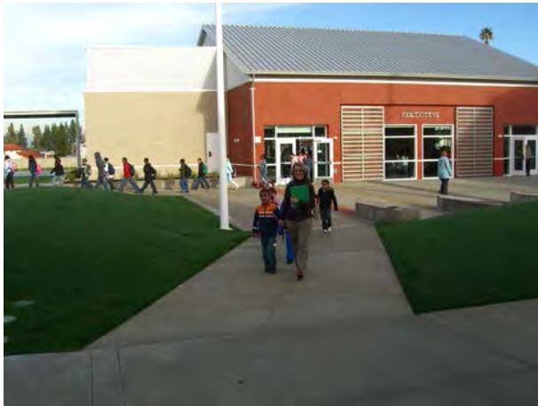
Kindergarten Classroom Finishes
