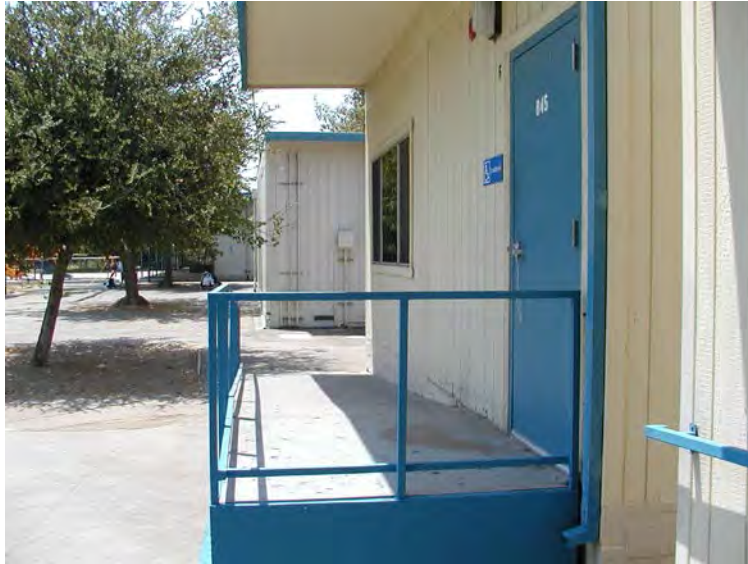
Relocated Portable Classroom
