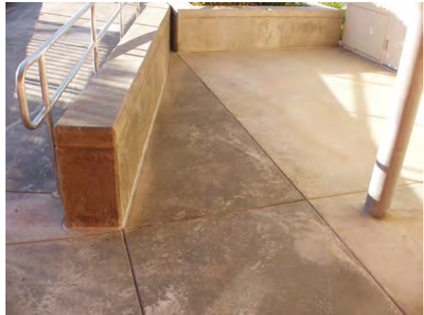
Completed Retaining Wall
