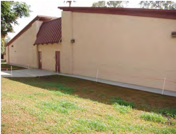
New Stucco at the Front of Library Building
