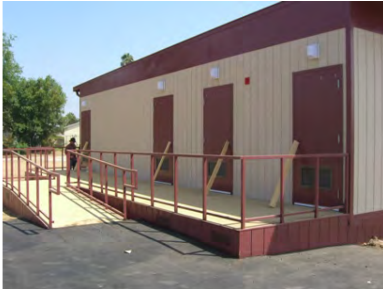
New Accessible Restroom
