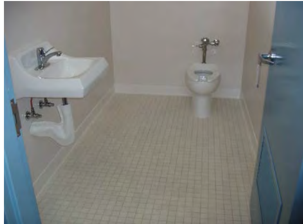
Completed Staff Restroom
