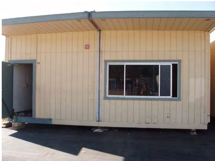
Portable being Relocated
