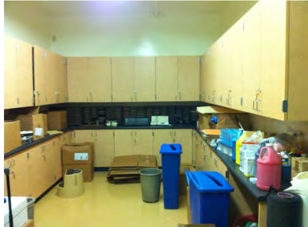
Completed Storage Room
