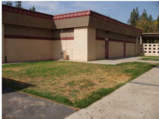
New Stucco at the Kitchen Wing
