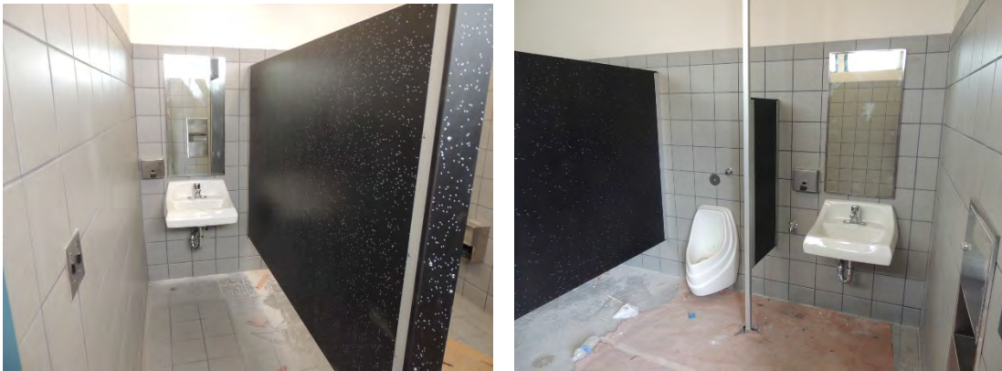
Monroe Elementary School Restroom – Completed restrooms
