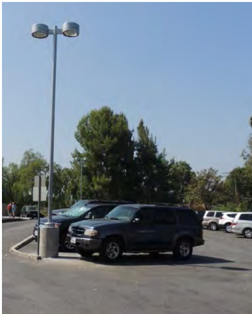
Completed Light Pole at Emerson Elementary School
