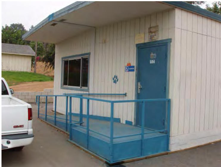
Relocated Portable Classroom
