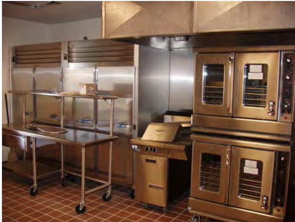
New Serving Kitchen Equipment
