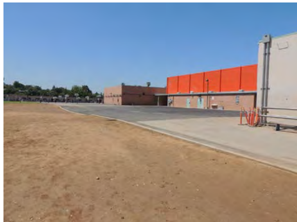
Demolished Old Pool Area
