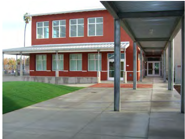
Administration Building at Library Walkway
