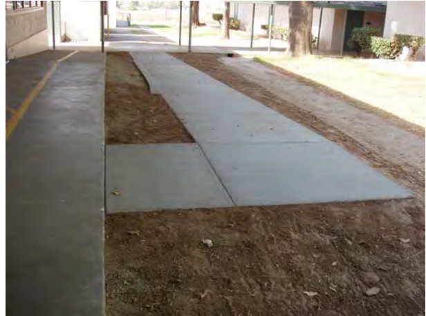
New Accessible Walkway
