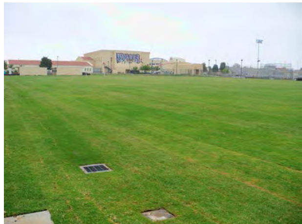
Completed Practice Field
