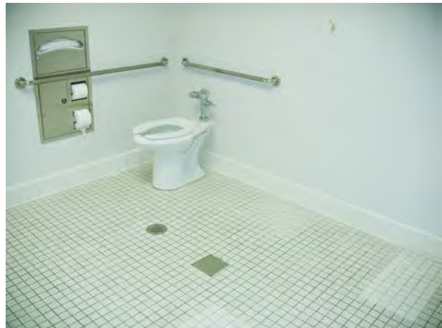
Remodeled accessible restroom
