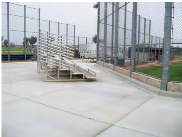
Completed Baseball Hardscape
