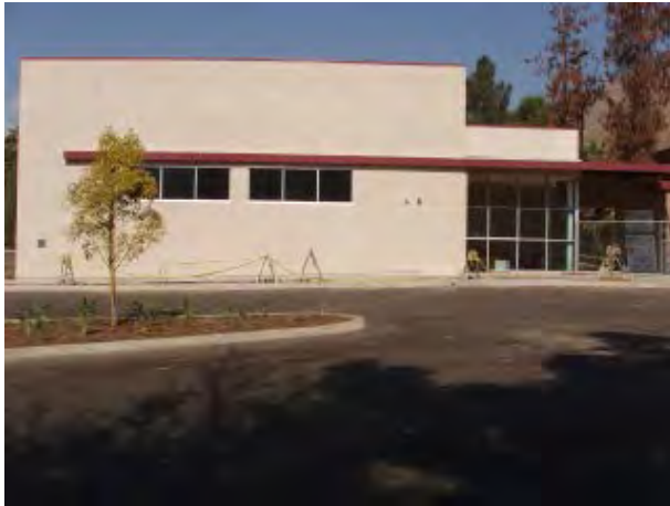
New Multi-purpose Room (MPR)
