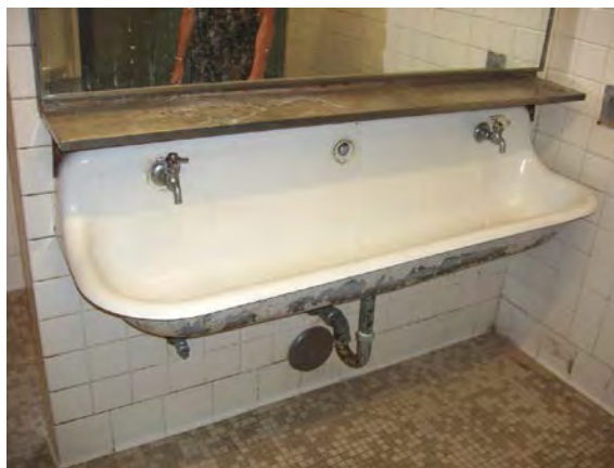
Existing restroom at Fremont Elementary
