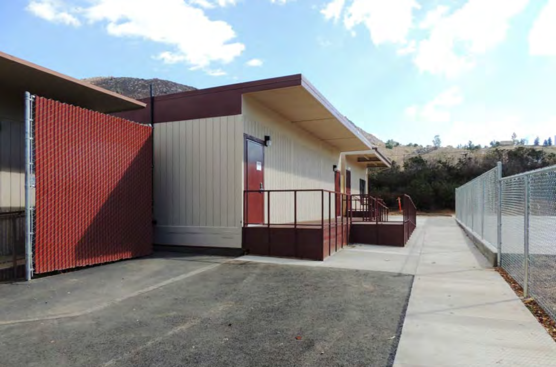
2015 Relocatable Classrooms in place
