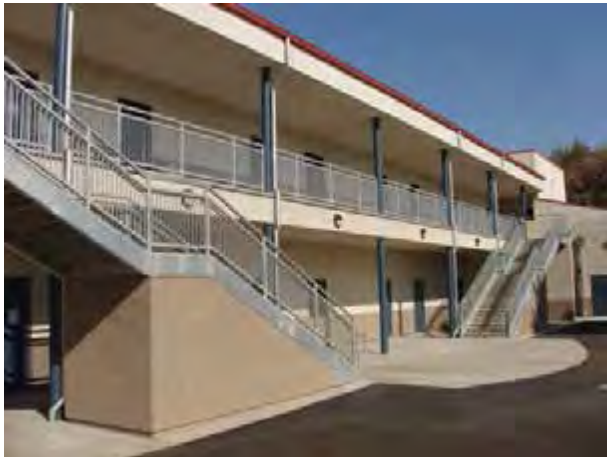
Classroom Portion of the New Wing
