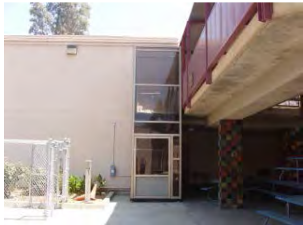
New Two-Story Wheelchair Lift
