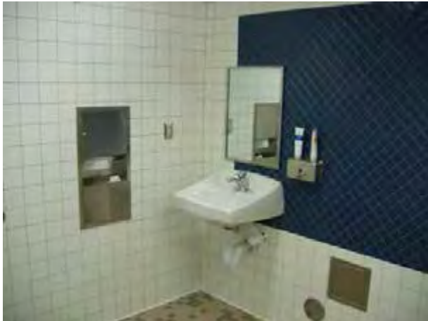
Completed Restroom Renovation
