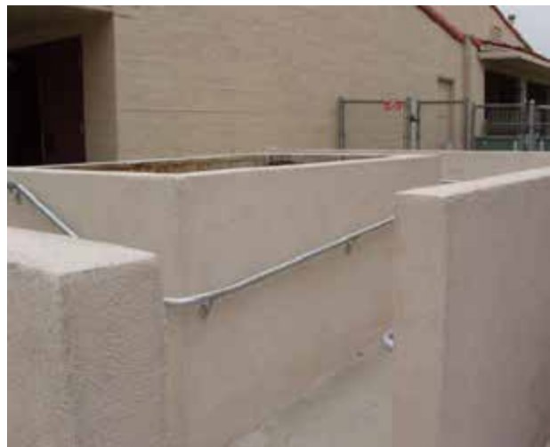
Outside MPR New ADA Ramp/Stairs
