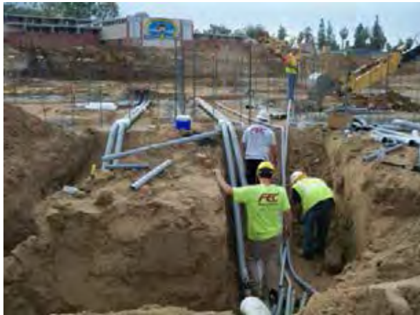
Installing Conduit for the Visitor's Concession Stand
