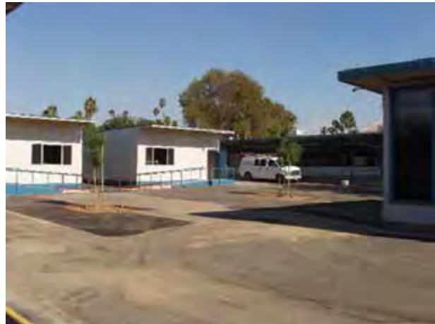
Completed New Portables
