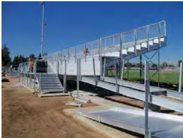
Track and Field Bleachers
