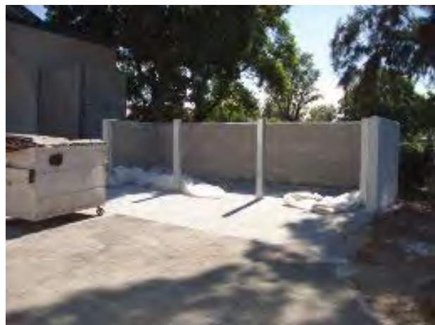
New Trash Enclosure
