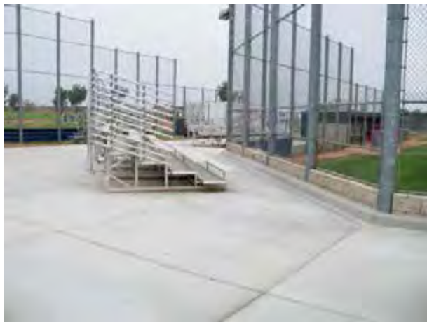
Completed Baseball Hardscape
