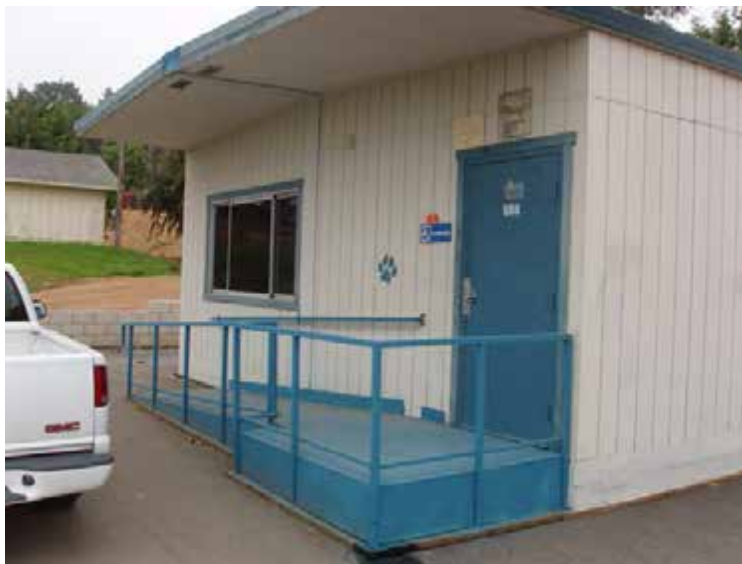
Relocated Portable Classroom
