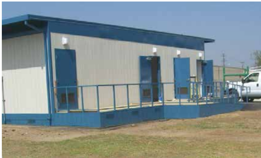
Completed Accessible Restroom
