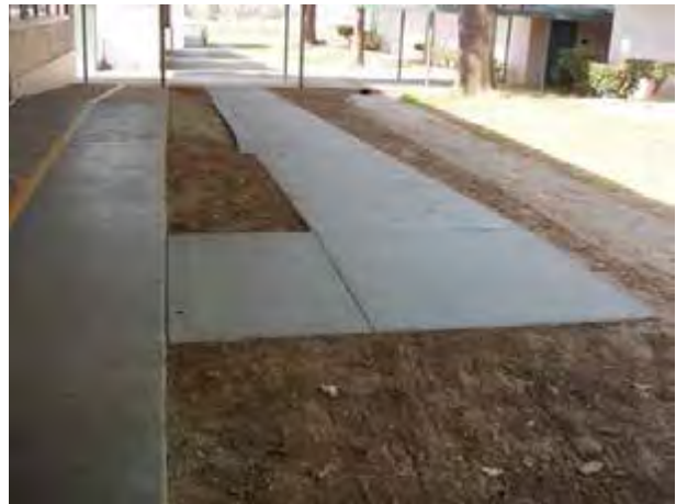
New Accessible Walkway
