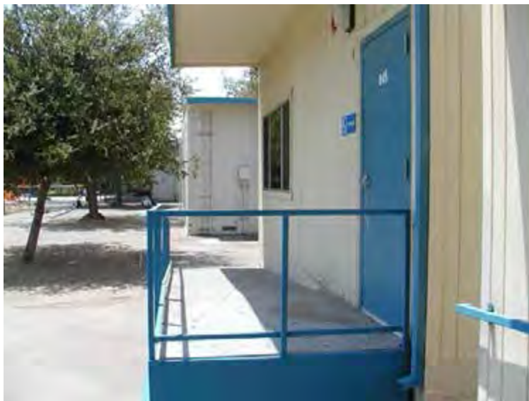
Relocated Portable Classroom
