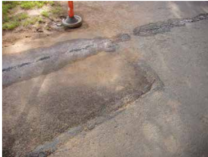
Completed Asphalt Addition
