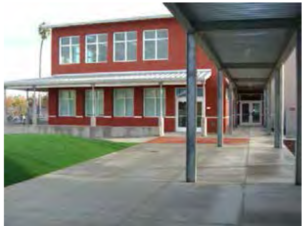
Administration Building at Library Walkway
