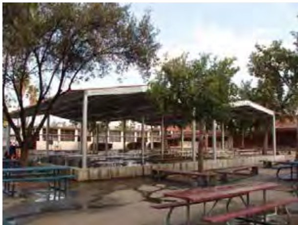
Completed Lunch Shelter
