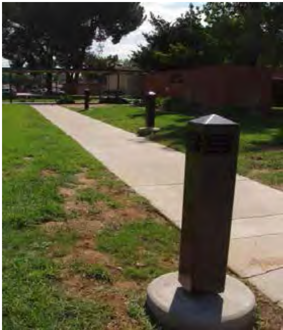
New Illuminated Walkway Bollards
