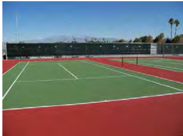
Completed Tennis Courts
