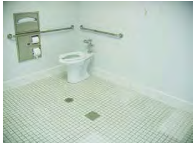
Remodeled accessible restroom
