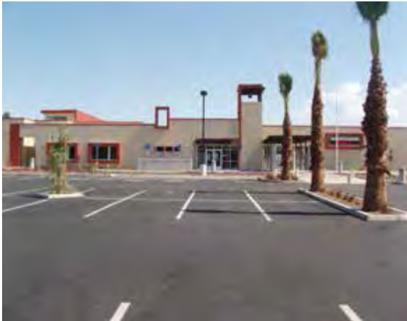
Front of New Administration/Library Building
