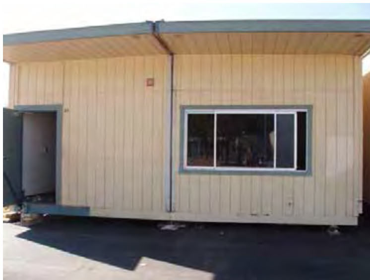
Portable being Relocated
