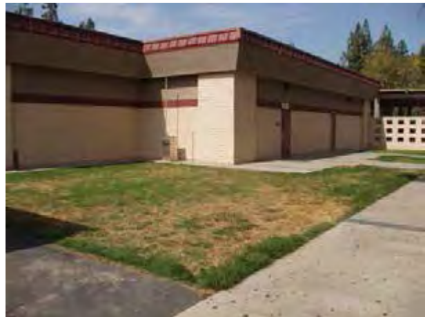
New Stucco at the Kitchen Wing
