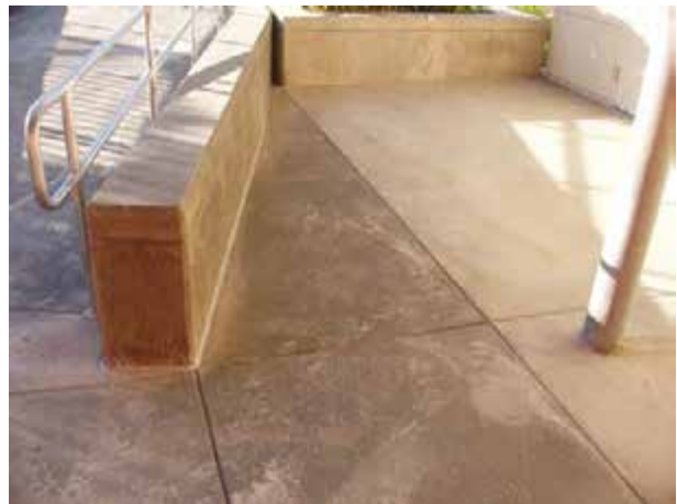
Completed Retaining Wall
