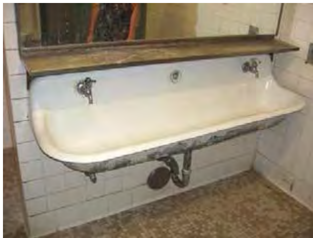
Existing Restroom at Fremont Elementary School
