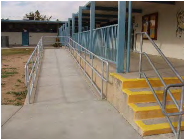
New Accessible Ramp
