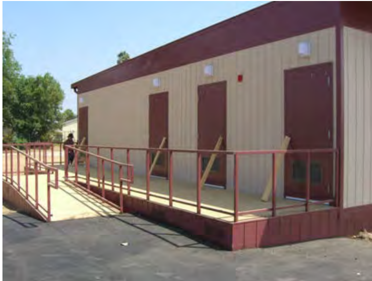
New Accessible Restroom
