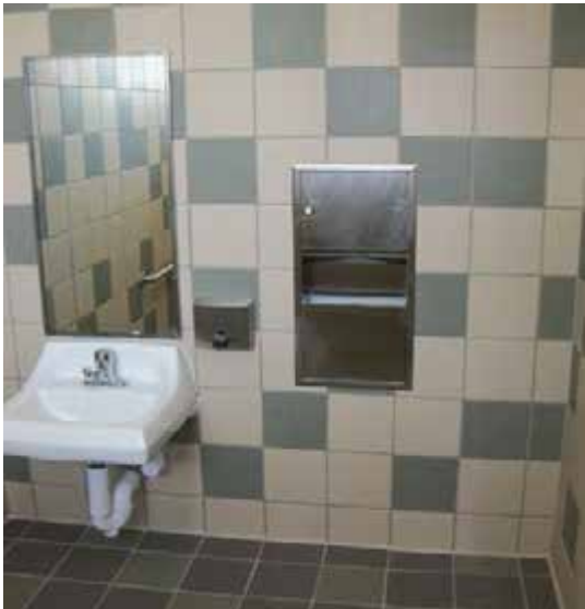
Completed Magnolia Restroom
