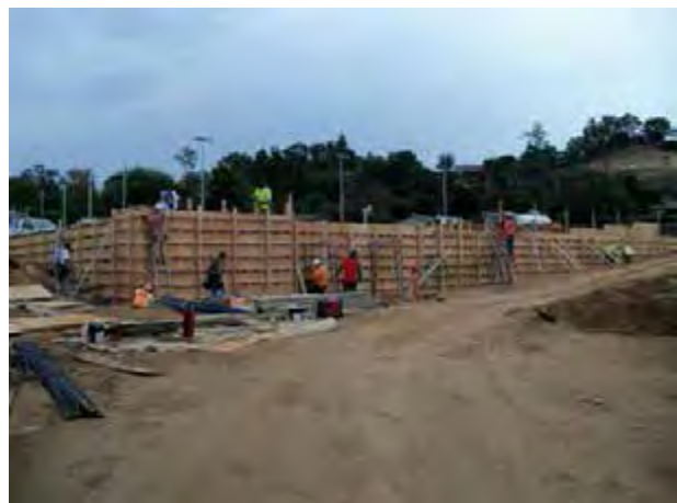
Track Retaining Wall
