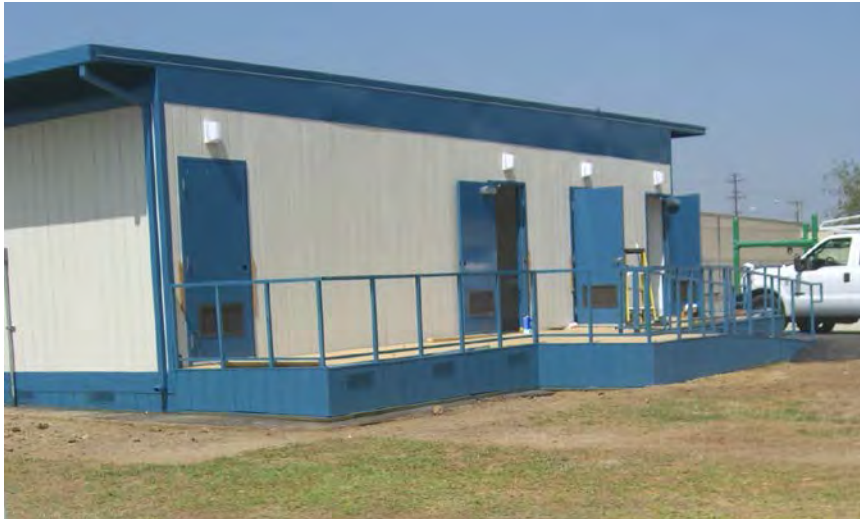
Completed Accessible Restroom
