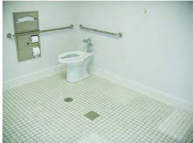
Remodeled accessible restroom
