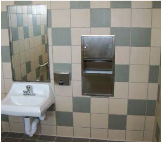
Completed Magnolia Restroom
