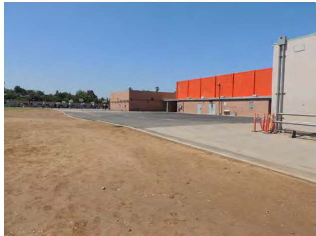
Demolished Old Pool Area
