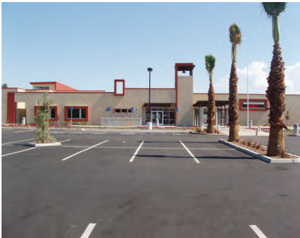
Front of New Administration/Library Building
