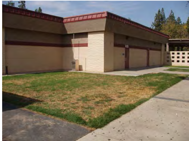
New Stucco at the Kitchen Wing
