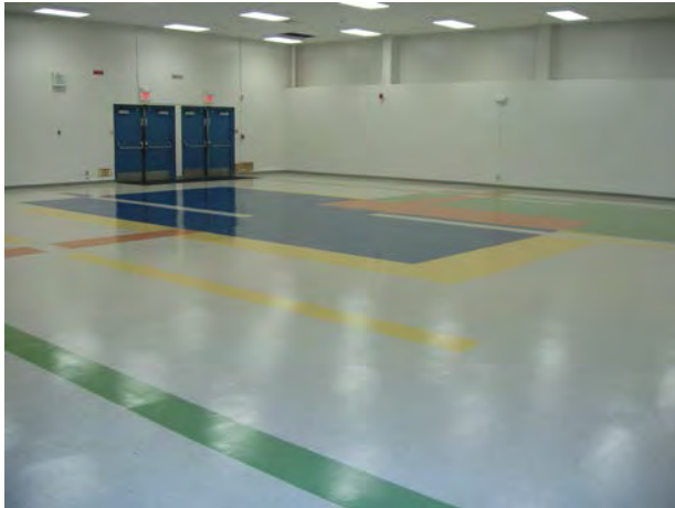
New floor for the MPR
