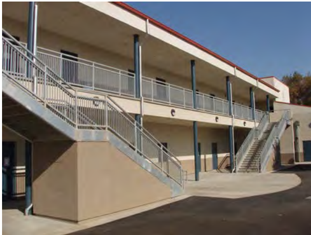
Classroom Portion of the New Wing
