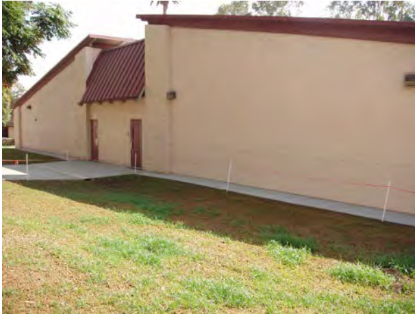
New Stucco at the Front of Library Building
