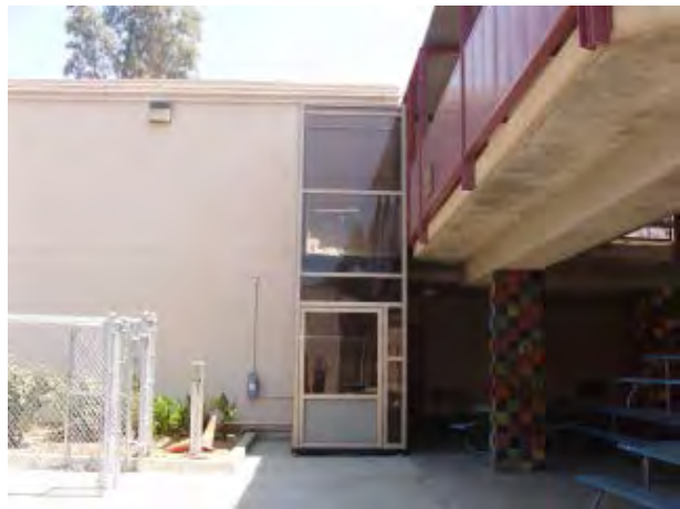
New Two-Story Wheelchair Lift
