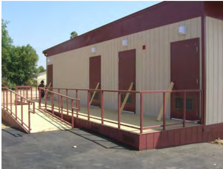
New Accessible Restroom
