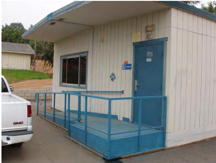
Relocated Portable Classroom
