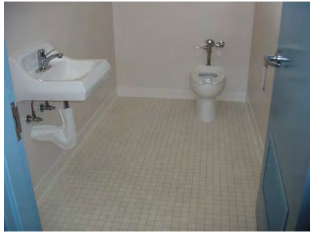
Completed Staff Restroom
