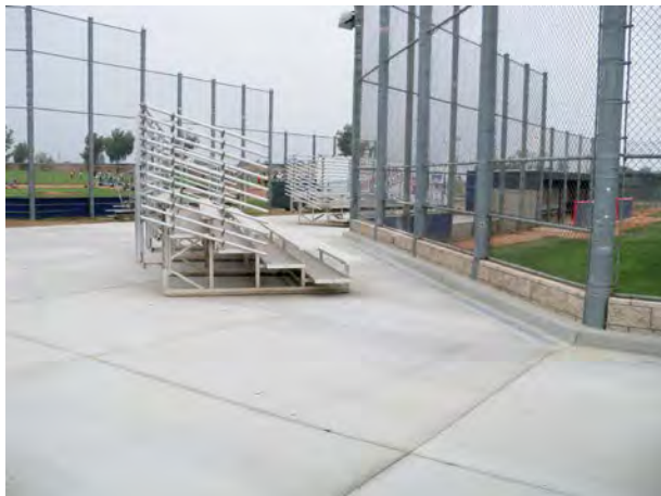
Completed Baseball Hardscape
