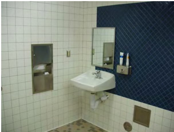
Completed Restroom Renovation
