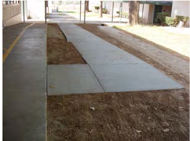
New Accessible Walkway
