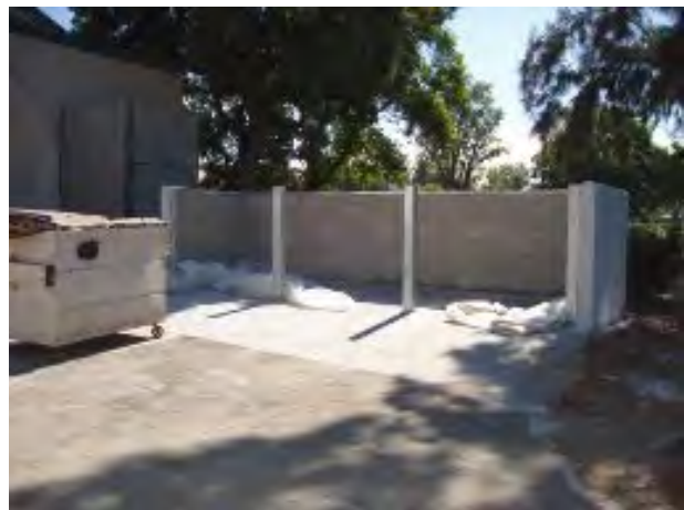
New Trash Enclosure
