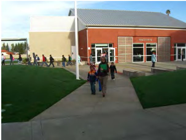
Kindergarten Classroom Finishes
