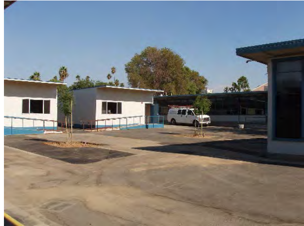
Completed New Portables
