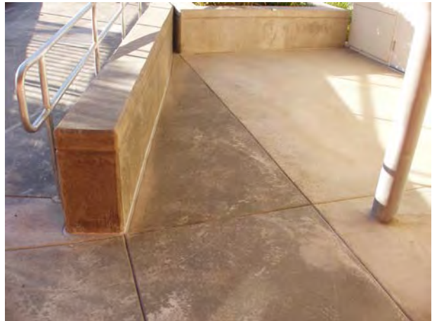
Completed Retaining Wall
