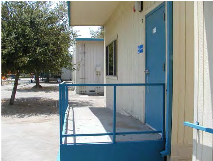
Relocated Portable Classroom
