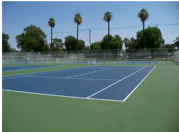
Completed Tennis Courts
