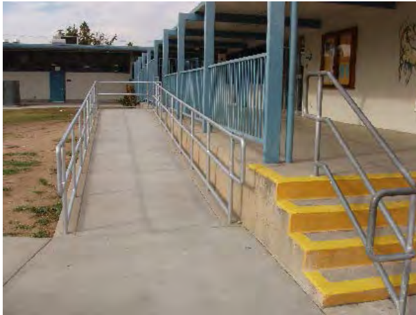
New Accessible Ramp
