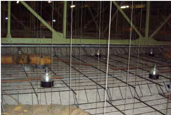
Suspended Plaster Ceiling
