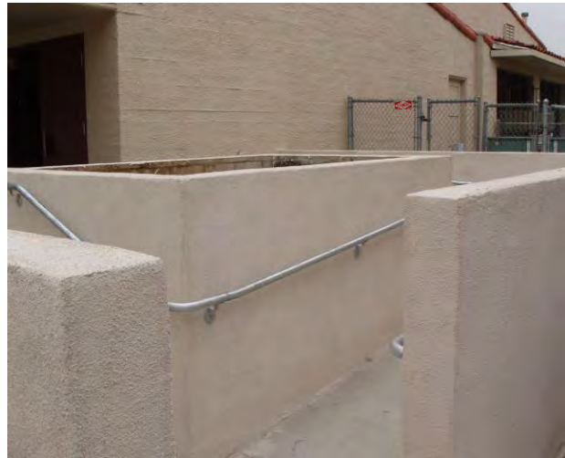
Outside MPR New ADA Ramp/Stairs
