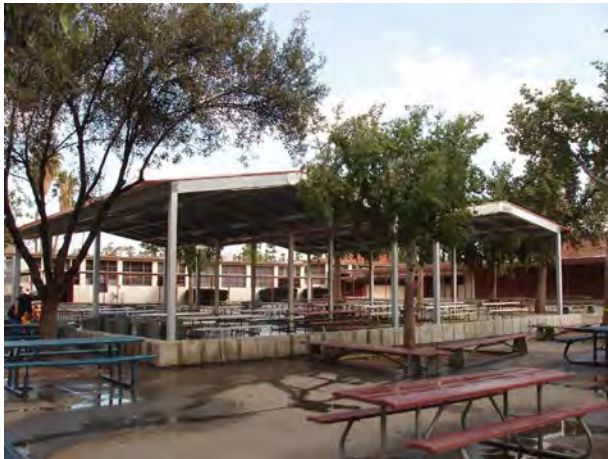
Completed Lunch Shelter
