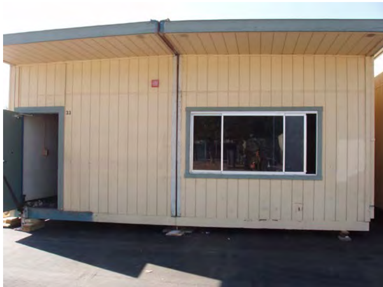
Portable being Relocated
