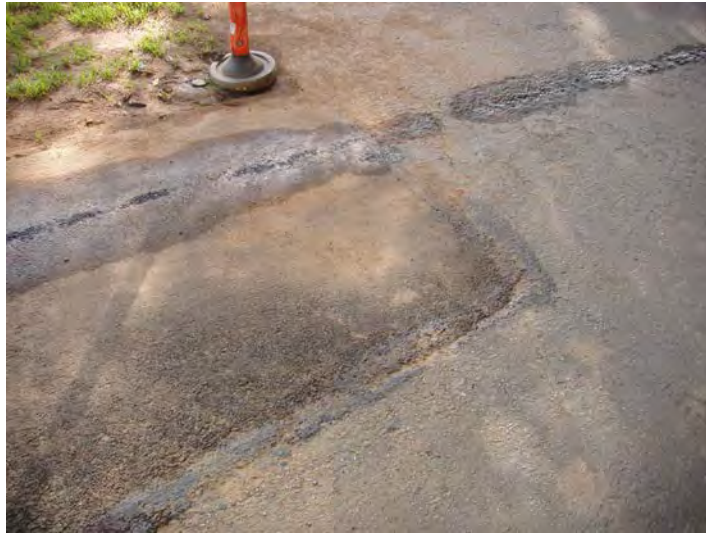
Completed Asphalt Addition
