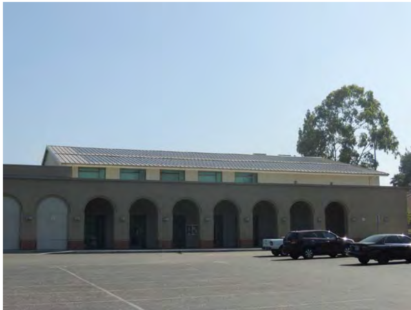
Existing condition; Central Middle School parking lot
