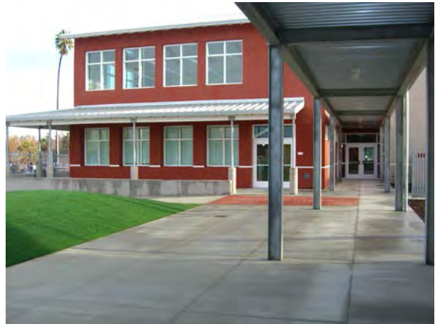
Administration Building at Library Walkway
