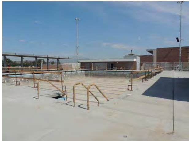
Pool Ready for Plaster
