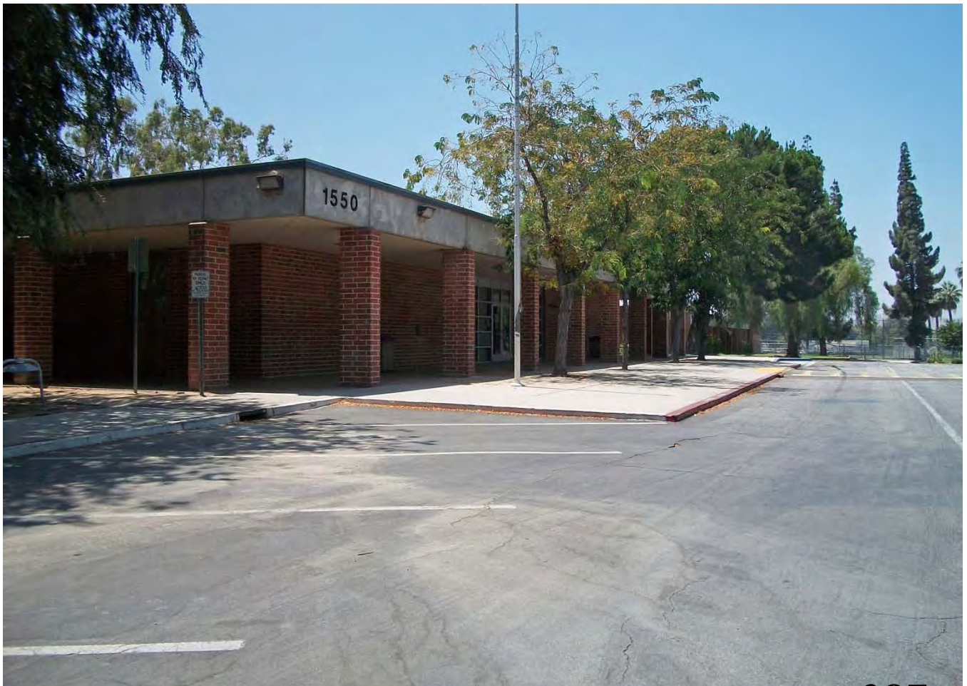
Overview of Administration Building (Southwest).
