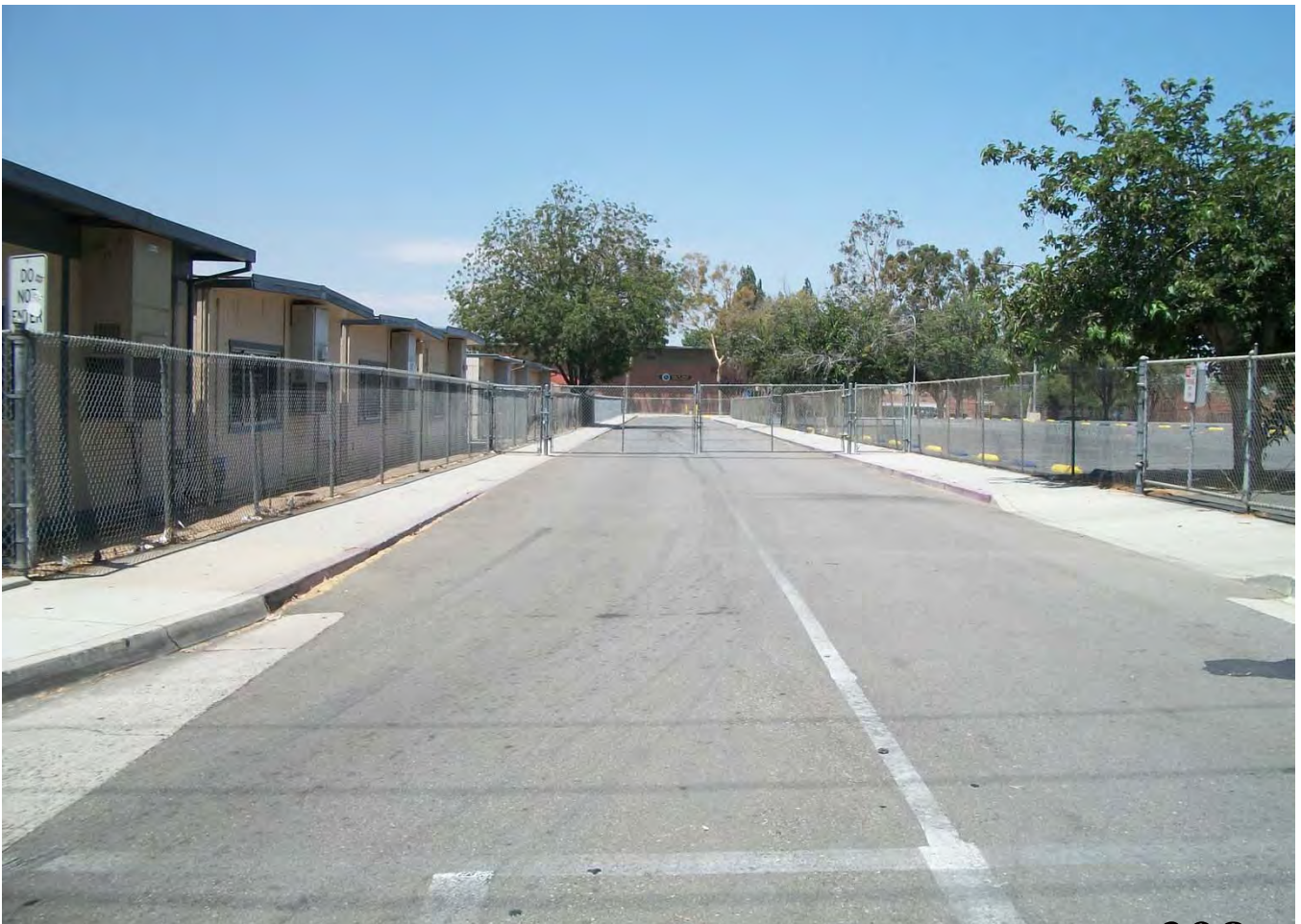
Access Road into Campus Near Portable Classrooms (North).
