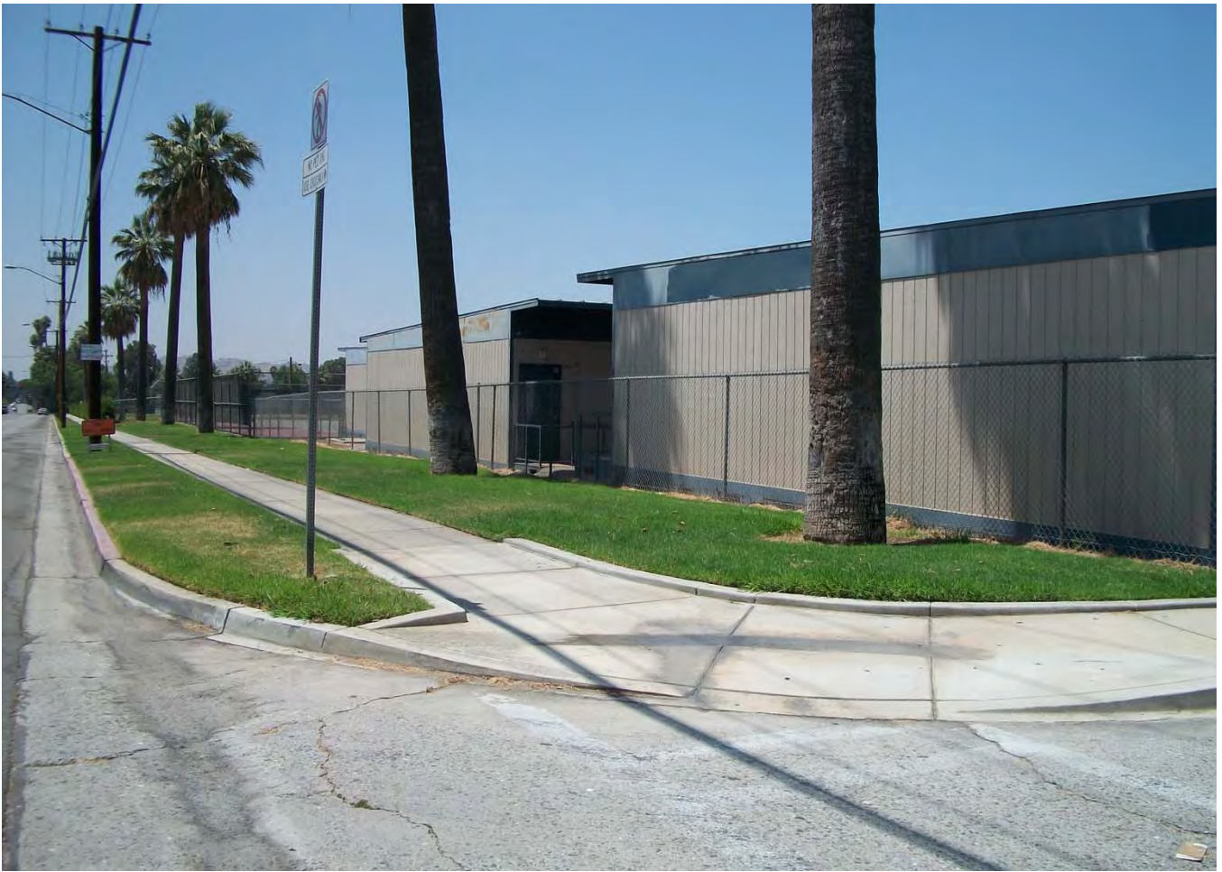
Portable Classrooms to East of Tennis Courts, from Linden Street (Northwest).
