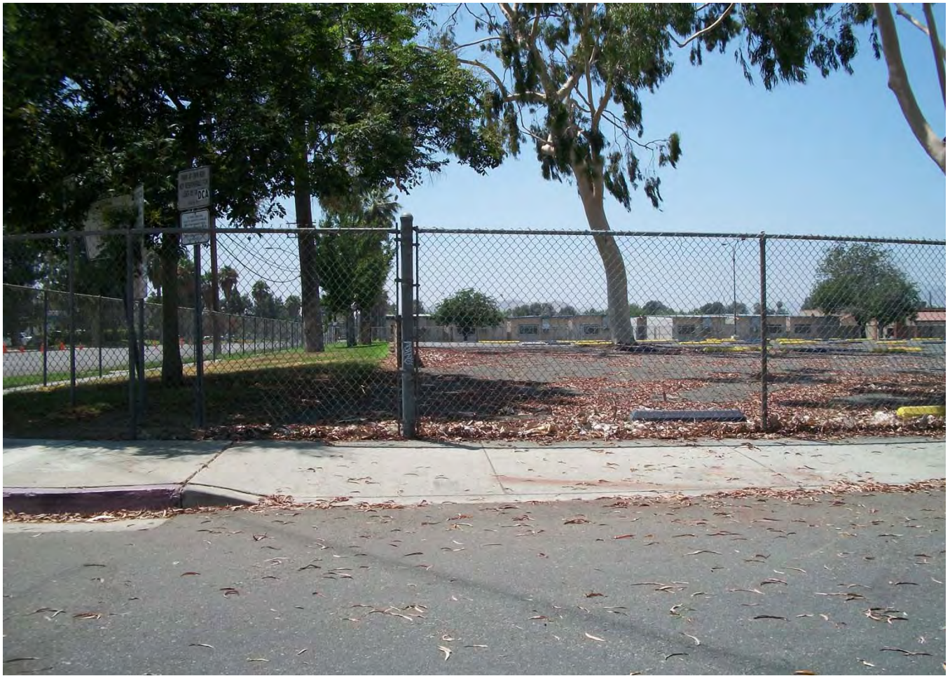
Southeast Corner of John W. North High School (West).
