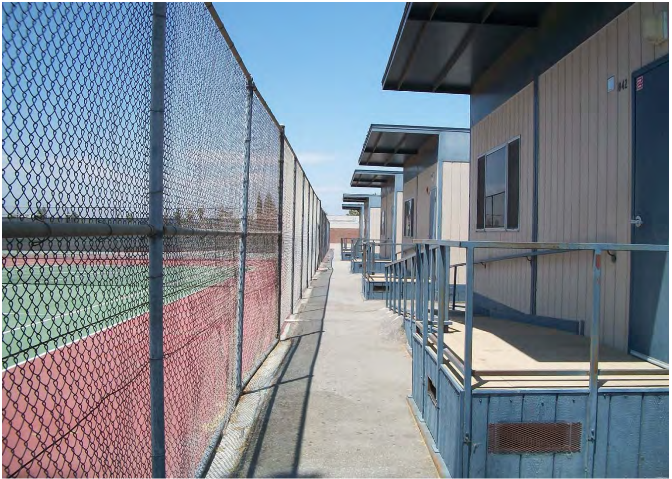
Area Between Tennis Courts and Portable Classrooms (North).
