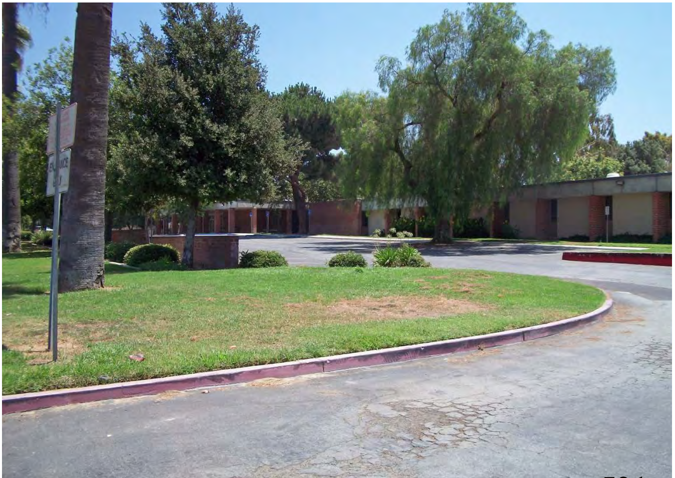
View from Entrance into Parking Lot Towards Administration and Classroom Building (Southeast).
