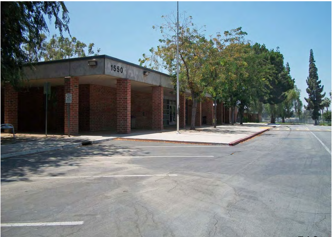
Overview of Administration Building (Southwest).
