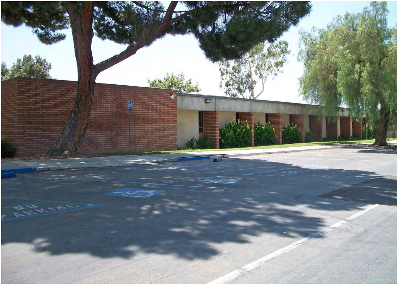
Classroom Building West of Administration Building (Southwest).
